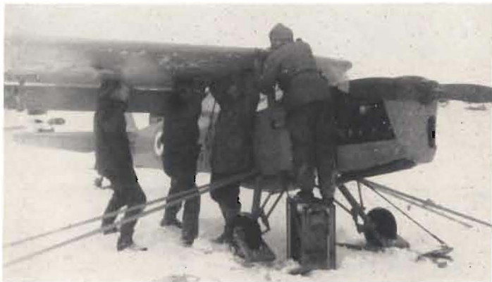
All hands joined together in assembling the second aircraft, which had remained crated throughout the voyage.
